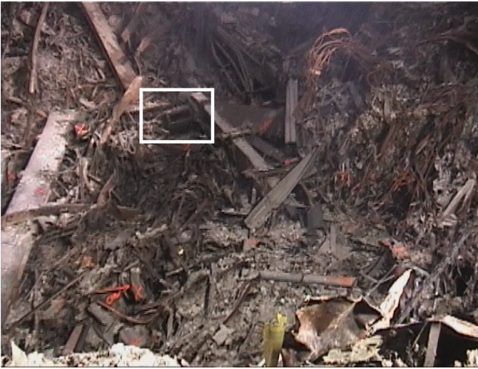
Fig. 4. WTC Tower 2 as an example of the physical challenges imposed by rubble: 0.5 x 0.3 m void opening searched by robot is shown within the box.
